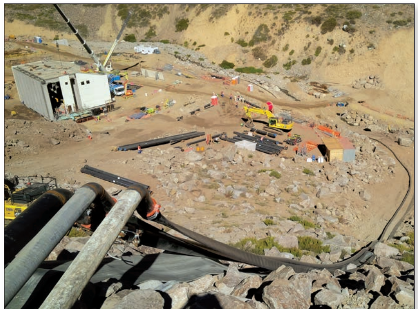
High pressure dewatering
