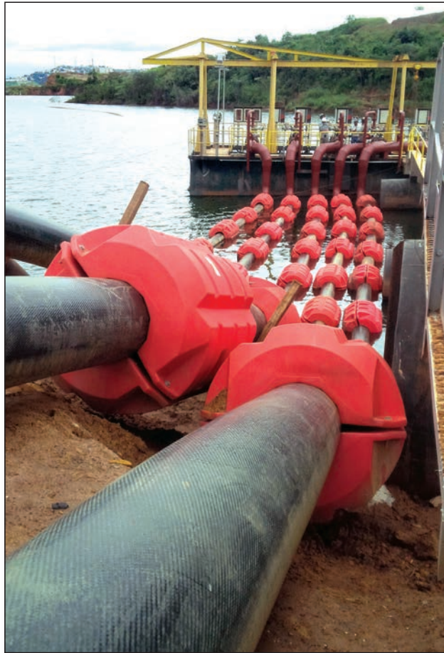
MINEFLEX on floating barge
