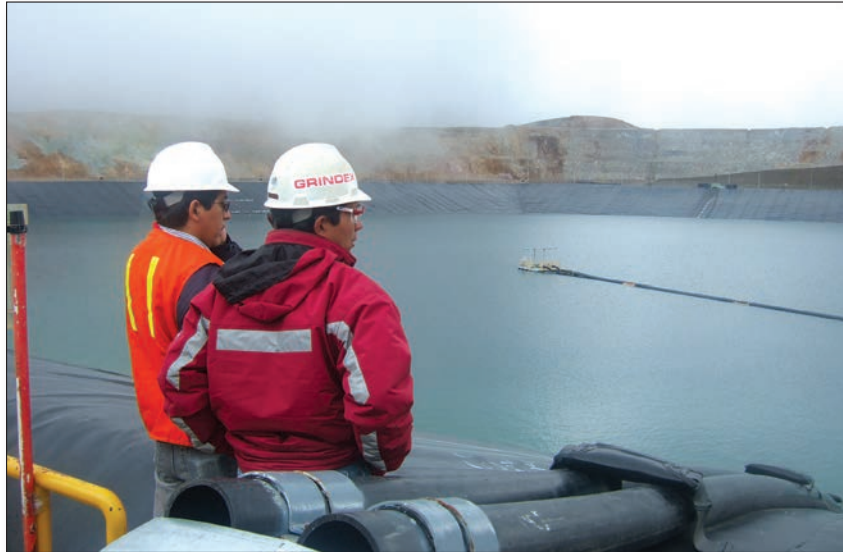
12" MINEFLEX on floating barge
