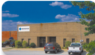
BENSHAW High Point EPC Division High Point, NC
